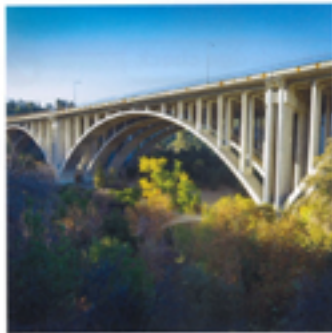
▲ A reinforced concrete bridge
