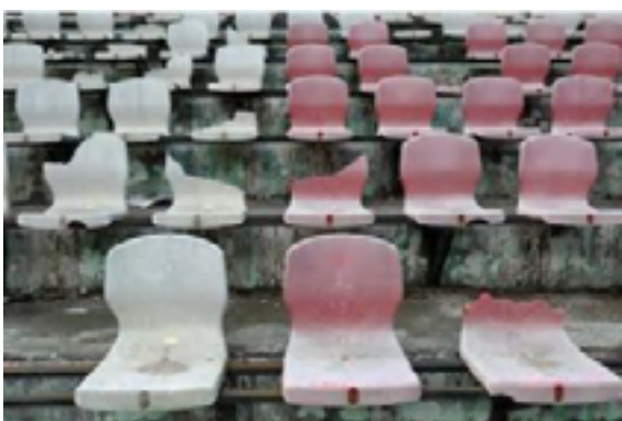
UV light can make plastic brittle and faded.
